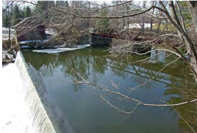
Mill River dam, 2009. Photograph C. Kellogg.
